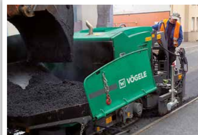
PAVING ASPHALT BETWEEN TRAMWAY TRACKS
