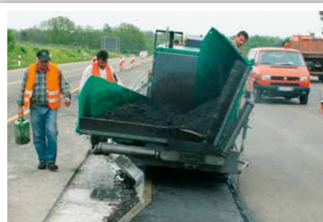
SURFACING MEDIAN STRIPS ON MOTORWAYS
