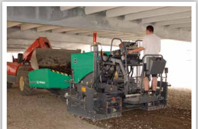
BUILDING THE BASE FOR PAVING SETTS
