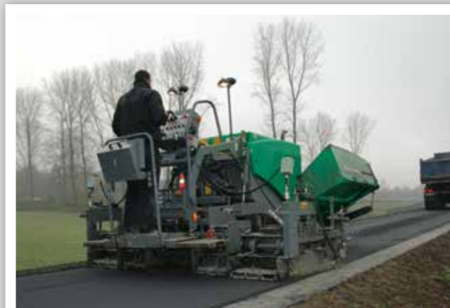
PAVING ASPHALT ON DAMS
