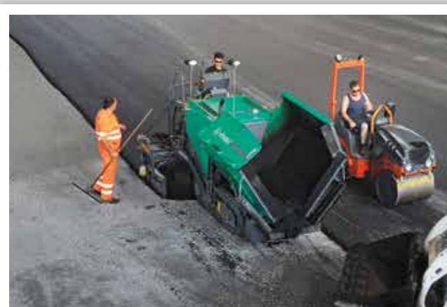
PAVING WORK IN SPORTS FACILITIES
