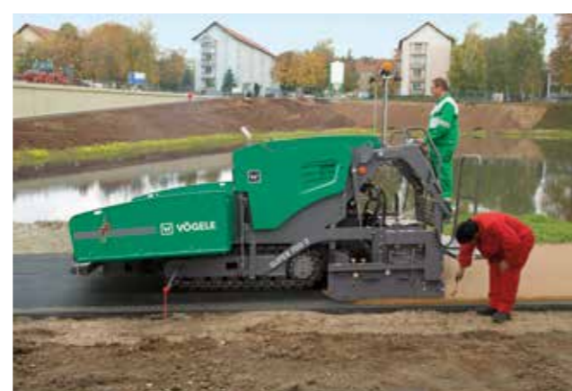
SURFACING CYCLE PATHS OR FOOTPATHS
