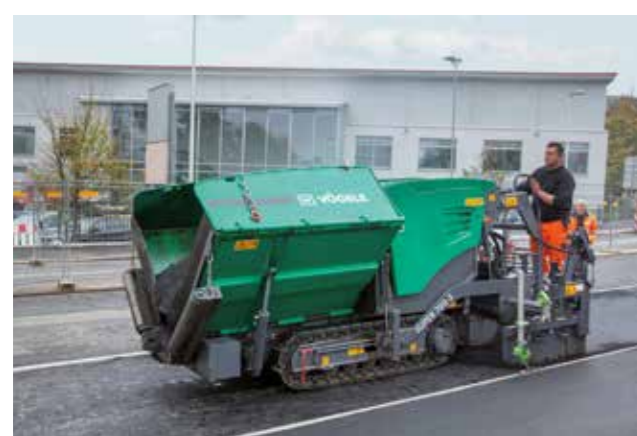
PAVEMENT REHABILITATION ON SMALL MUNICIPAL ROADS
