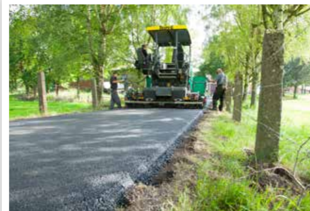
PAVEMENT REHABILITATION ON ACCESS ROADS
