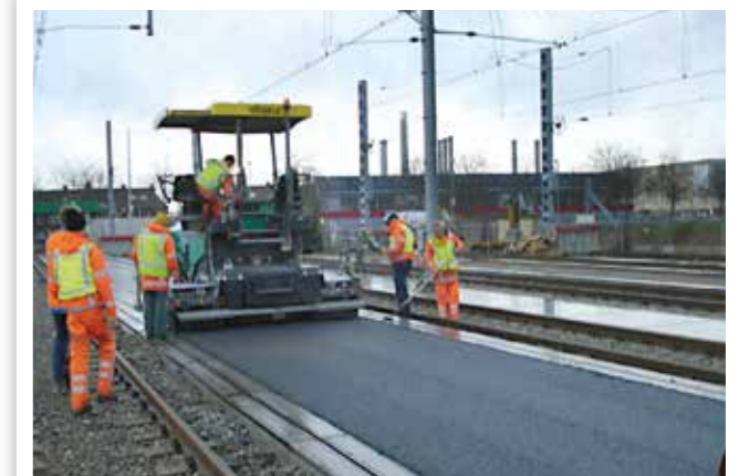
ASPHALT PAVING ON RAILWAY PLATFORMS
