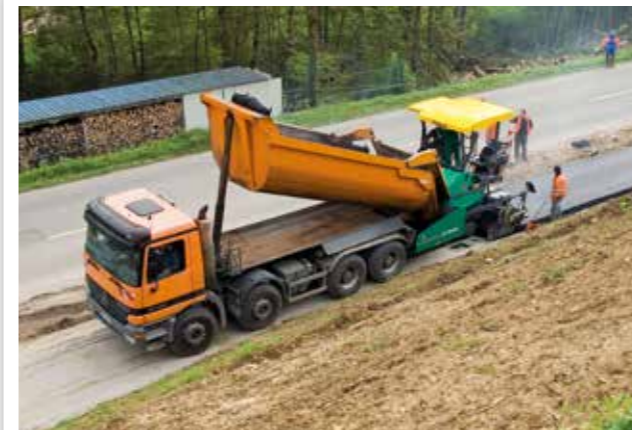
ASPHALT PAVING ON COMBINED FOOT AND CYCLE PATHS
