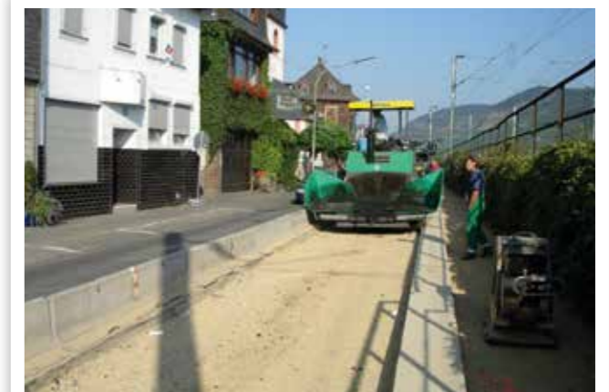
PAVEMENT REHABILITATION ON MUNICIPAL ROADS
