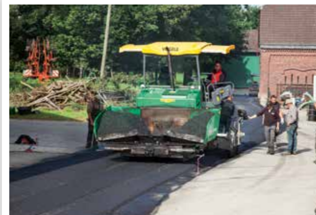
ASPHALT PAVING ON SURFACES USED FOR INDUSTRIAL PURPOSES
