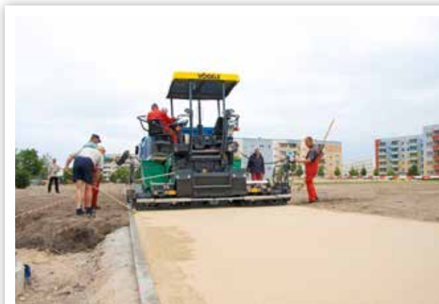
PAVEMENT REHABILITATION ON ACCESS ROADS
