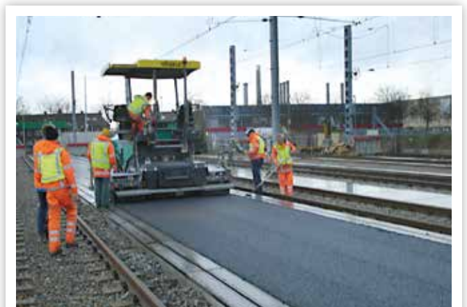
ASPHALT PAVING ON RAILWAY PLATFORMS
