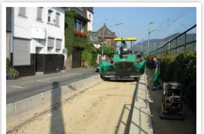
PAVEMENT REHABILITATION ON MUNICIPAL ROADS
