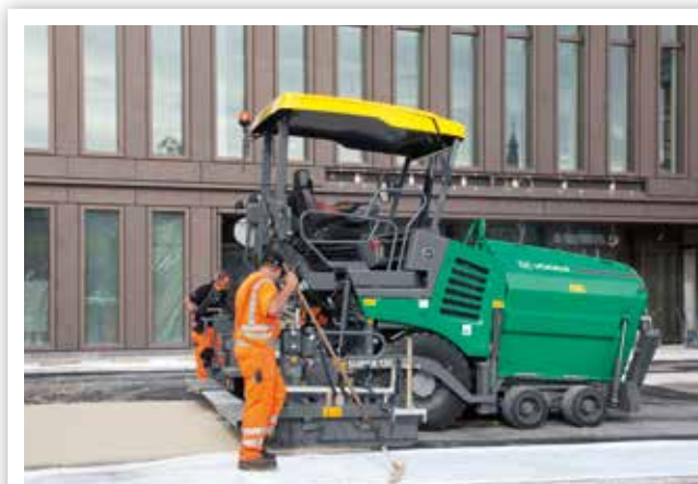
ASPHALT PAVING ON COMMERCIAL SITES
