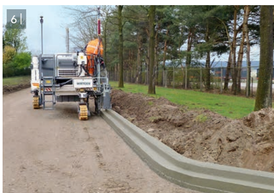
7 | Producing a slot drain to ensure rain-water drainage.
