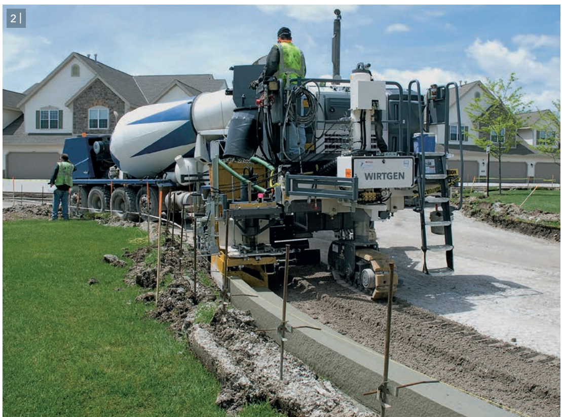
2 | No problem for the SP 15/SP 15i: paving radii to pin-point accuracy.
