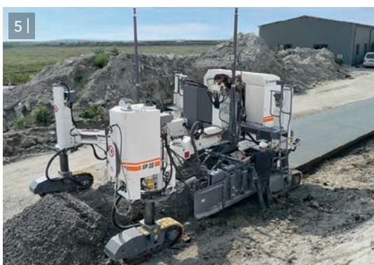
4 | Paving tracks for an agricultural road.
